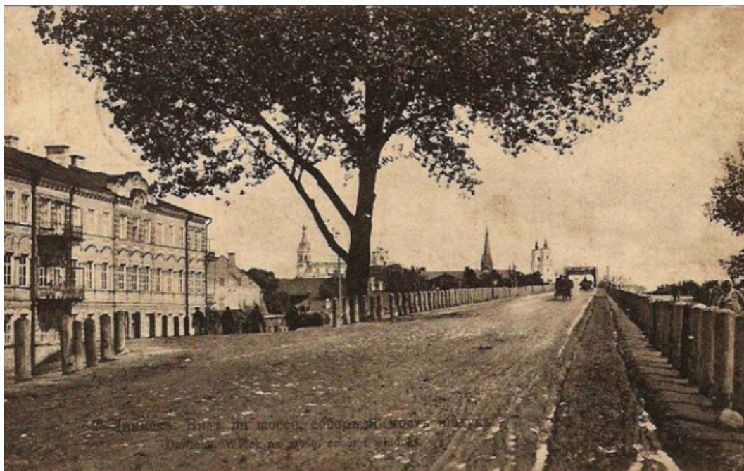
Daugavpils. View of the highway, cathedral and bridge in the distance
